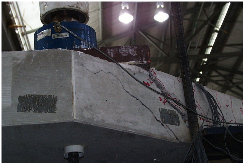
Figure 6-19 Failure of breakback UTSE overhang, side view of slab, facing south
