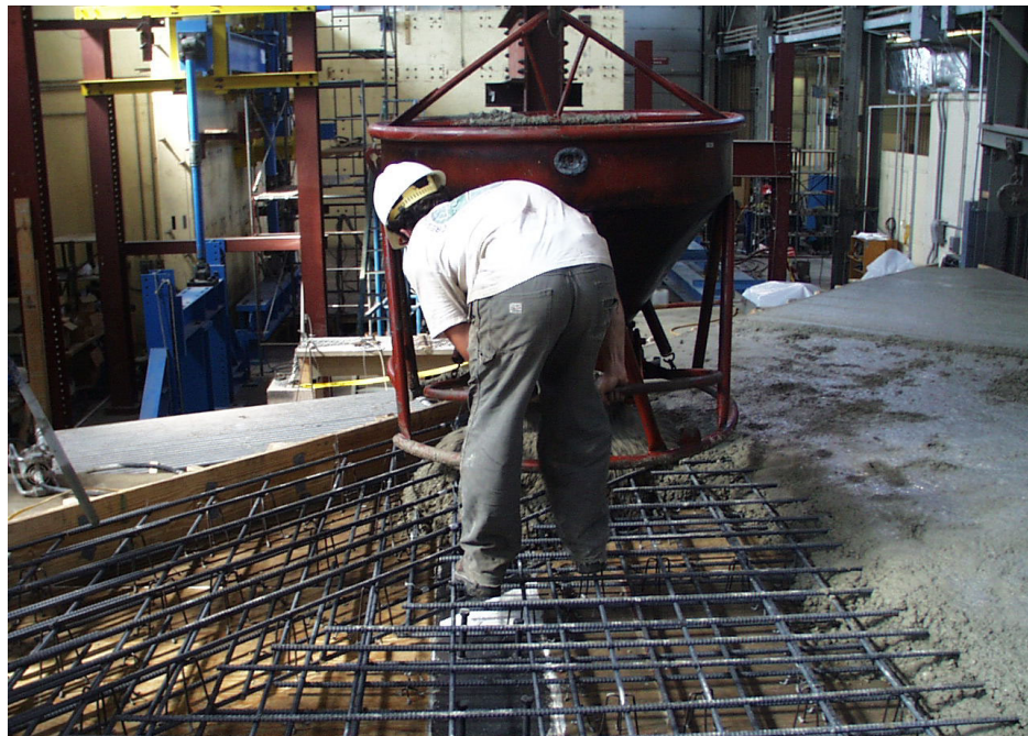
Figure 4-3 Pouring the slab
