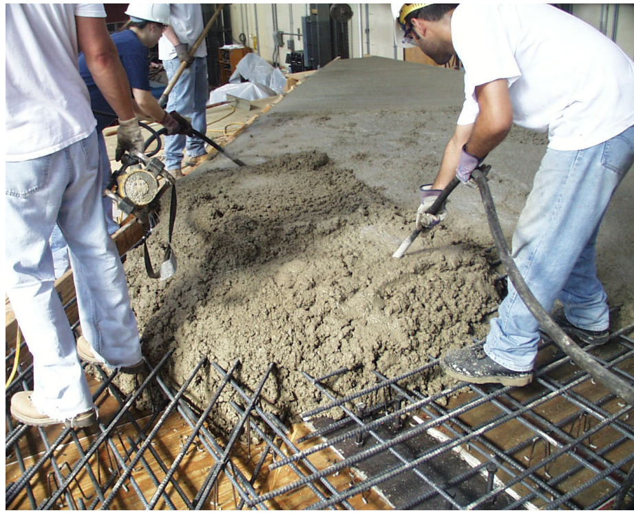
Figure 4-4 Vibrating concrete
