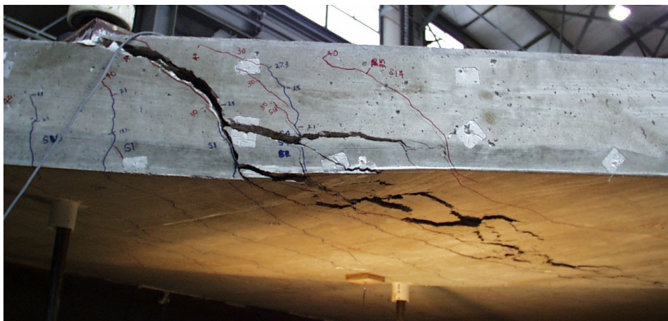
Figure 5-39 Failure surface at side of slab, facing north
