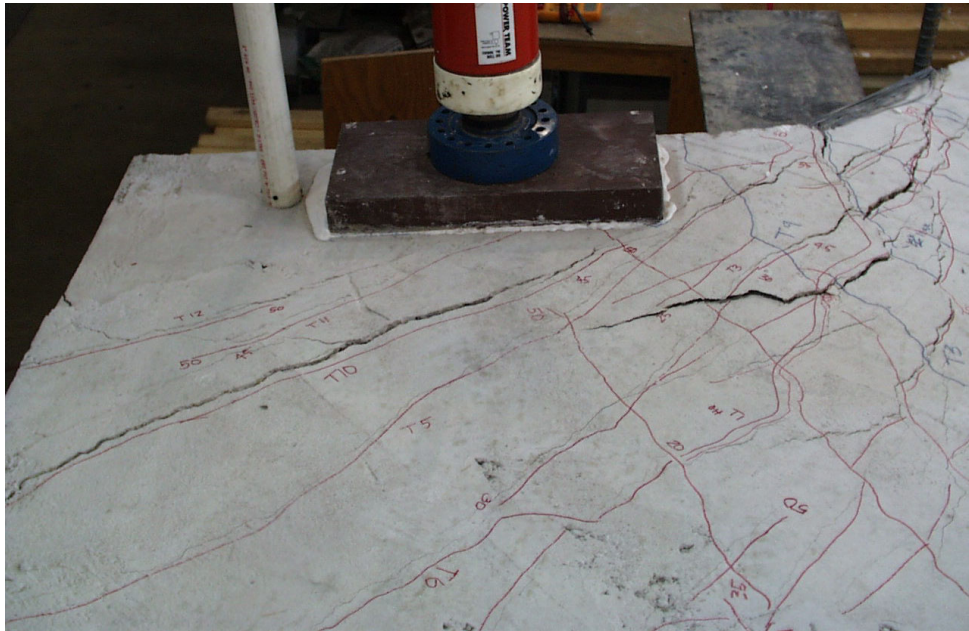
Figure 6-34 Failure of simulated 0° skew UTSE overhang, top view of slab, facing north
