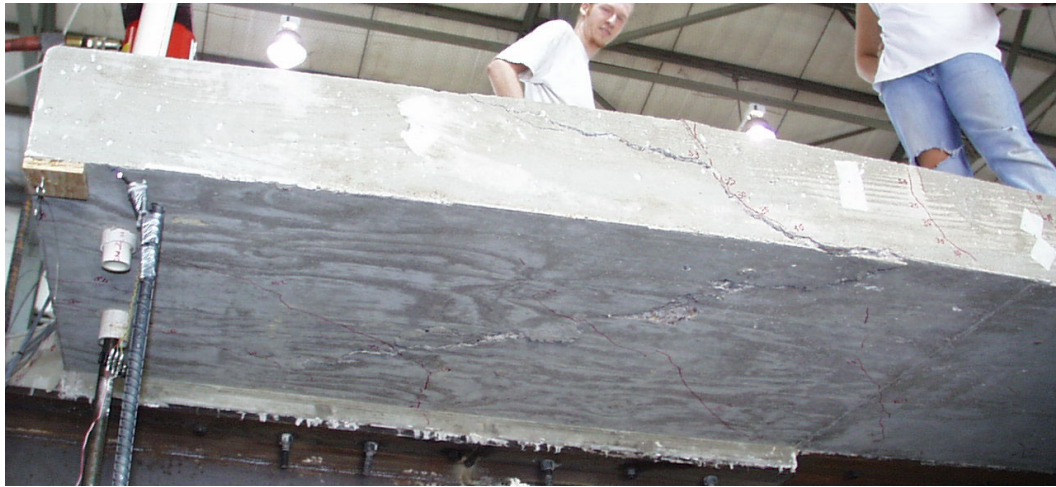
Figure 6-28 Failure of simulated 0° skew IBTS overhang, bottom view of slab facing west
