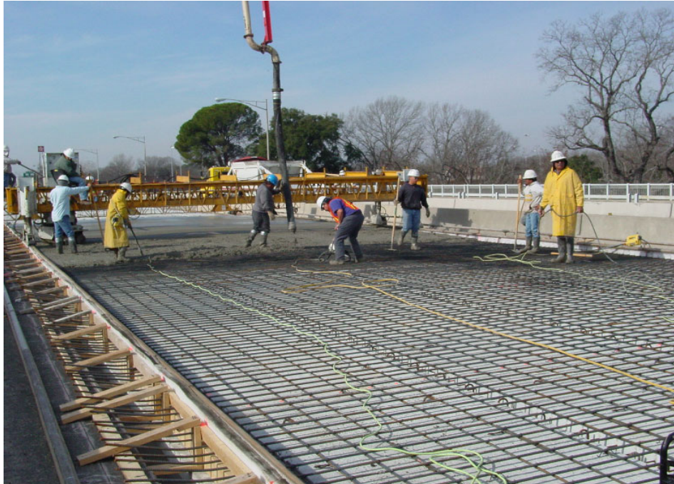
Figure 1-5: Placing of concrete in the field
