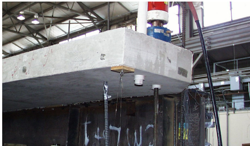
Figure 6-20 Failure of breakback UTSE overhang, bottom view of slab, facing southwest
