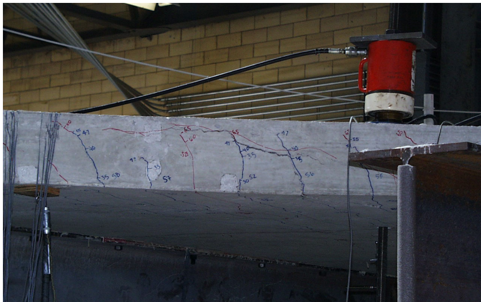
Figure 5-29 Exterior bay failure surface at side of slab, facing south
