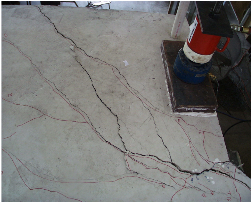
Figure 6-26 Failure of simulated 0° skew ITBS overhang, top view of slab, facing east
