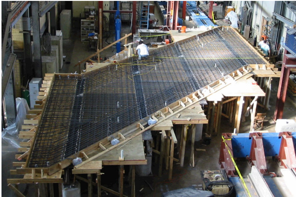
Figure 4-2 Forms before pouring
